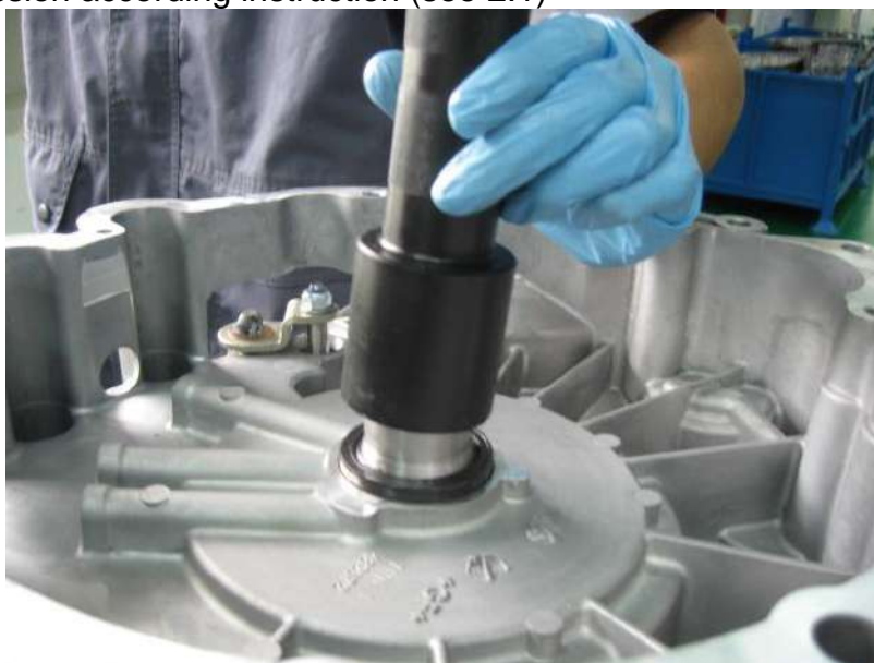
Fig. 3-4: Installing seal by special stamp (480130)
